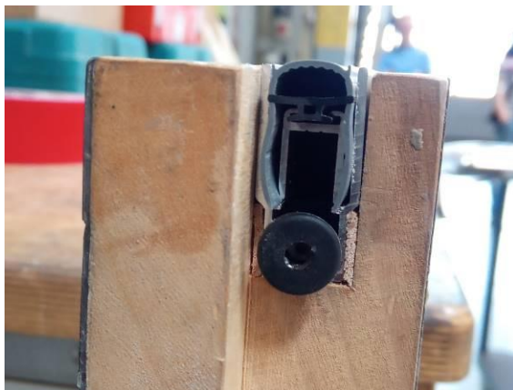
Fig. 4 Photo of floor seal in door leaf section
