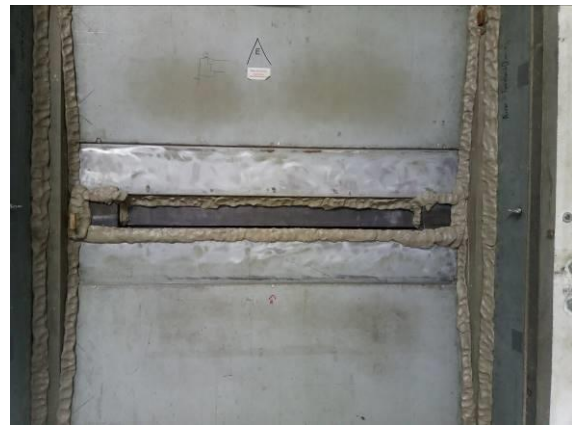
View from receiving room
